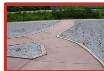
透水性高炉水砕スラグ舗装
